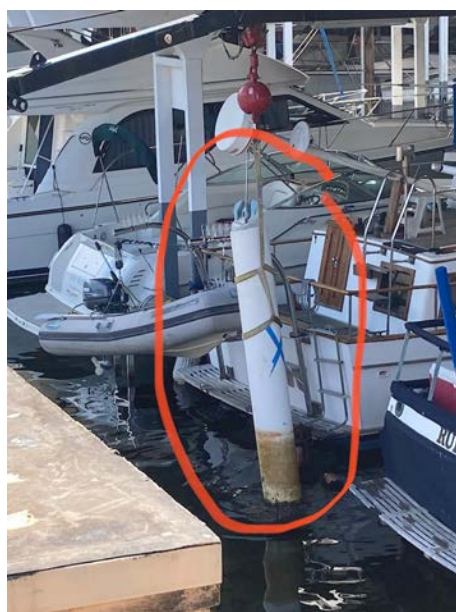
Some Center Piles listing Port of Starboard
