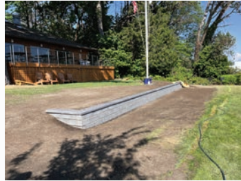
Outstation Wall Make Over
